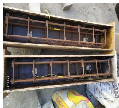
Fig. 10. Beams with reinforcement
