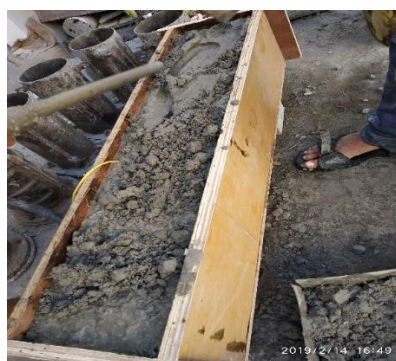
Fig. 11. The casting of beams with reinforcement
