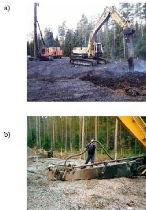
Fig. 14. Type of equipment for mixing soil by the mass method (a); the mixing hose and mixing unit on the ground surface (b)
