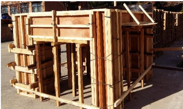
Photo 1: Form of concrete structures
