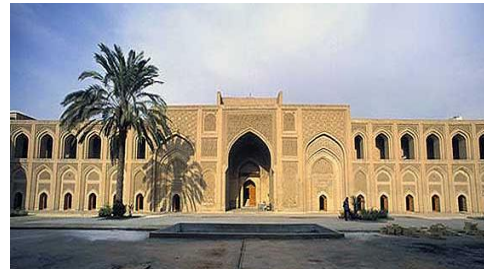
Fig. 2 Al-Mustansiriya school with its Islamic Architecture Style – Source: https://www.al-monitor.com
