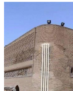
Fig. 3 Façade ruins by using method of fixing rain pipes in the heritage ones- source: Authors
