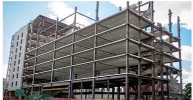
Figure 1: Steel Framed Structure
