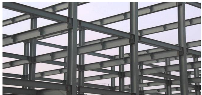
Figure 2: Different Steel Sections in Buildings
