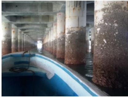
Fig.1 Examples of Pile Corrosion
