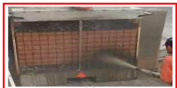
Fig3-shotcrete method.
