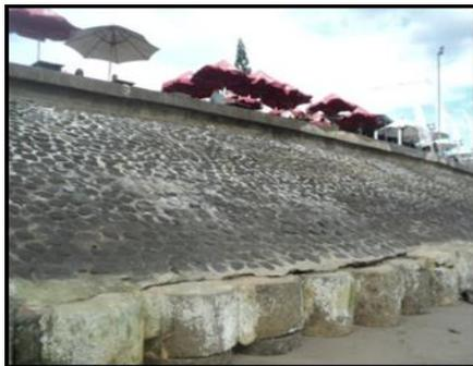
Figure 2. Seawall Crumbling on Canggü Beach, Bali, Indonesia (Nalarsih, 2016)
