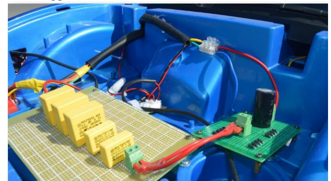
Fig 6: Secondary Capacitor bank & High Frequency Rectifier
