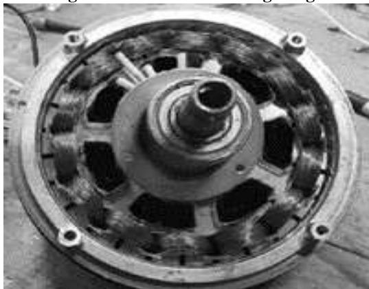
Fig.7 Defect 1 rotor winding gray image
