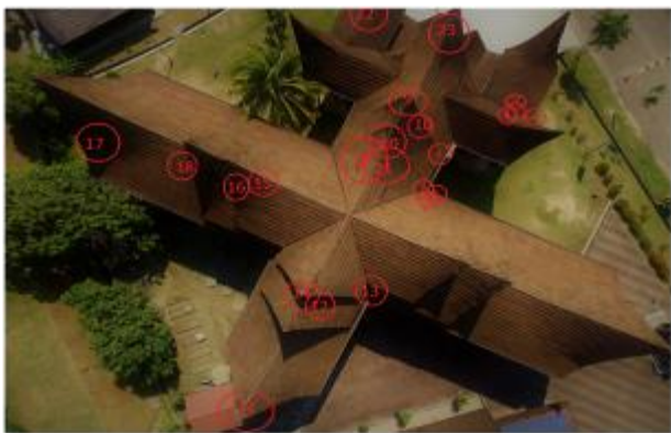
Figure VII: The location of defects for roof
