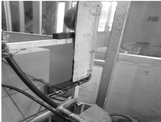
Figure 2 LPG inlet with control valves and Diesel-DEE fuel tank
