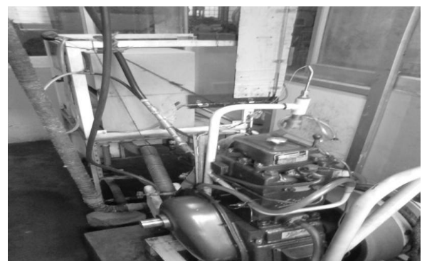
Figure 1 Engine overall view
