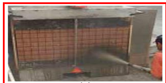
Fig3-shotcrete method.
