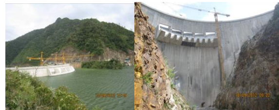
Fig. 9. Nam Chien arch dam (upstream and downstream)
