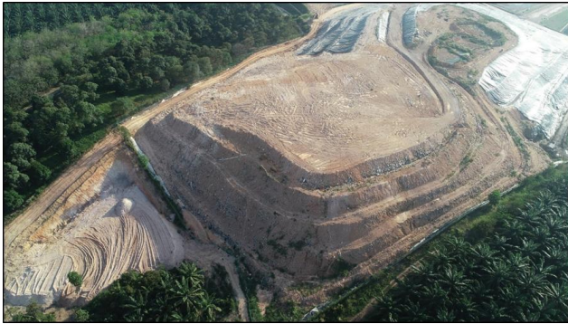
Fig. 2. Slope reconstruction in Sg. Udang, Melaka
