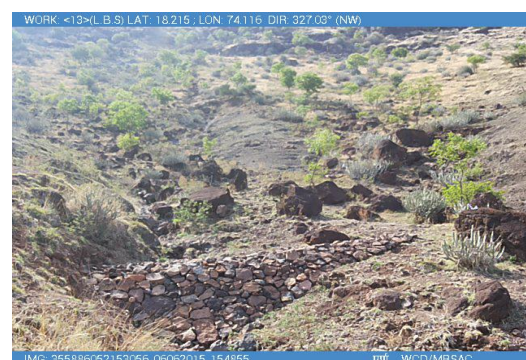
Fig. 9. Gabion Bund in Pingori
