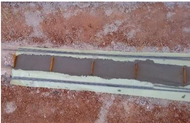
Fig. 2. Preparation of precast segments
