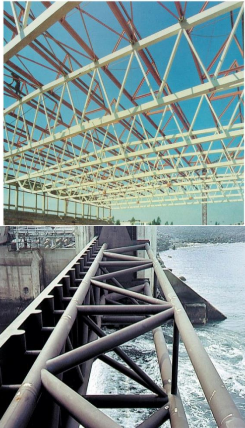
Fig. 5 Examples of Hollow Steel Section
