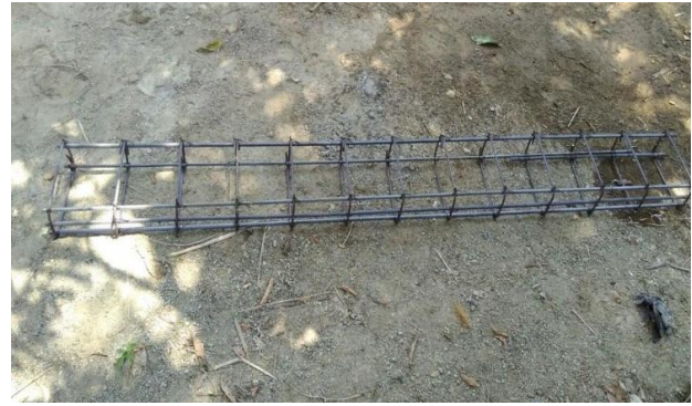
Fig.2 Reinforcement cage of beam
