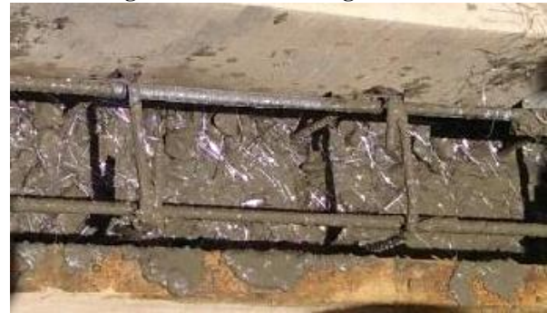
Fig.3 Beam concreting with steel fibre
