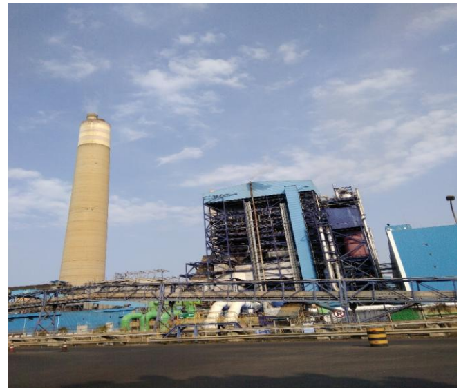
Figure 1. Steam power plant of PT POMI Paiton
