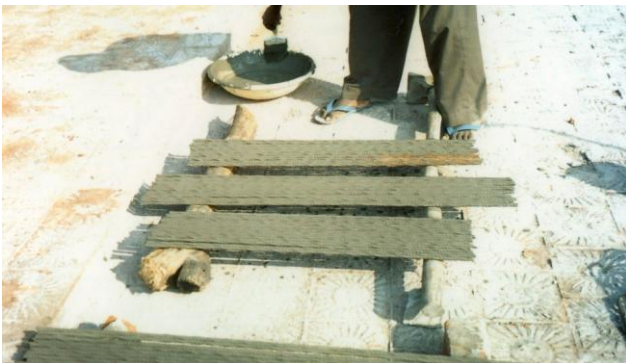
Fig. 3.Cement polymer anticorrosive coating in progress
