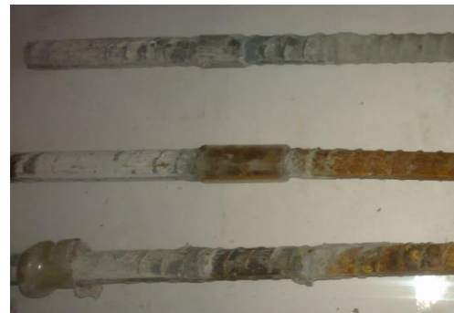
Fig. 12. Close View of Rebar after Pull out Test The close view of rebar after pull out experiment in this we can clearly find the unbond fill of 20mm has been inserted.
