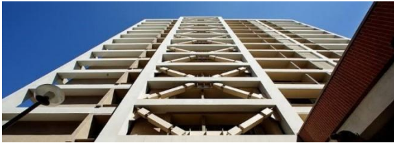
Figure-2: Cross Bracings
