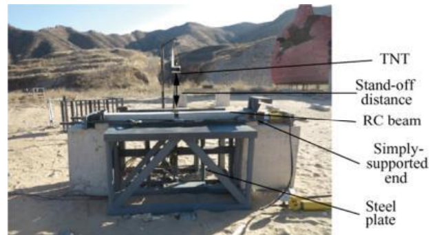
Fig. 9. Field Blast test set up of RC beams and columns, Liu et al (2018)
