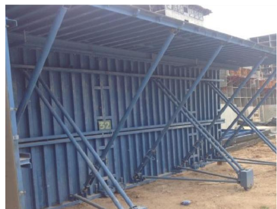
Figure 8. A few glimpses of the site at Rampally
