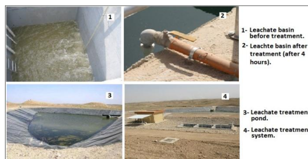
Fig. 6. Leachate treatment system at Kirkuk sanitary[29]
