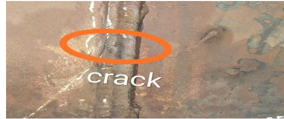
Fig. 13, a: linear cracks located on specimen surface.
