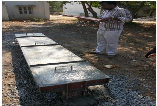
Fig 2. Beam mould after pouring of concrete
