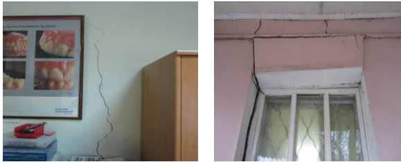
Fig. 4. Examples of photo-fixation of cracks (position on the scheme of the building)
