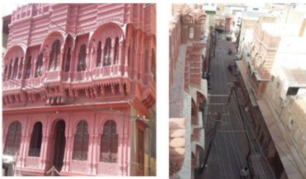
Figure 4: Haveli Façade and Shadade Street
