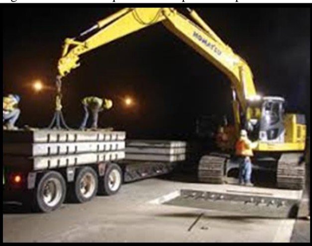
Image 3: Heavy machine on site
