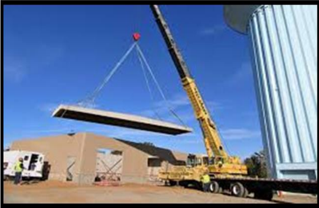
Image 1: Heavy machine lifting precast panel
