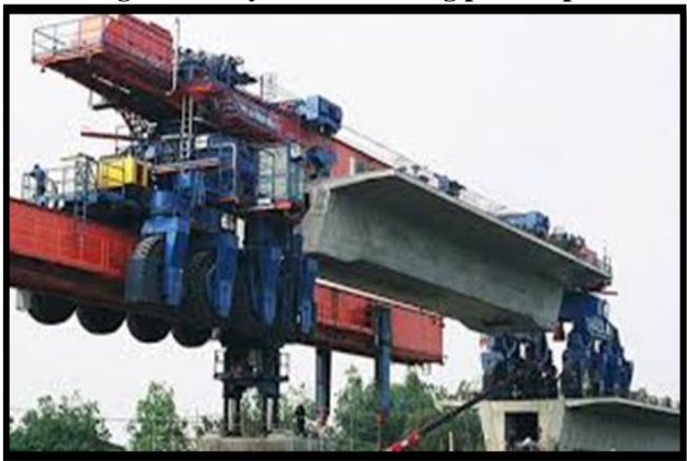
Image 2: Heavy machine lifting precast member
