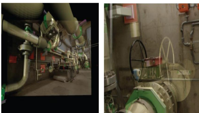
Figure 16: AR used for discrepancy analysis in industrial facilities. Courtesy of Nassir Navab [21]
