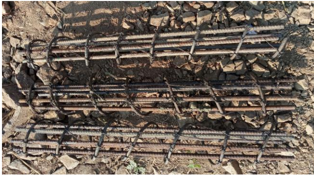
Fig.6 spirally shape stirrups @ 110 mm c/c spacing
