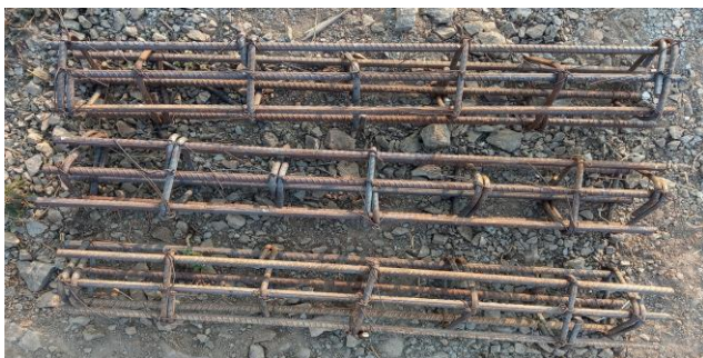
Fig.9 Triangular shape stirrups @ 110 mm c/c spacing
