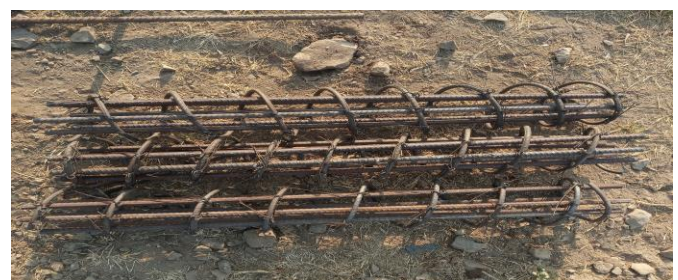
Fig.5 spirally shape stirrups @90 mm c/c spacing
