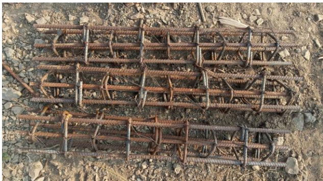
Fig.7 Triangular shape stirrups @ 70 mm c/c spacing
