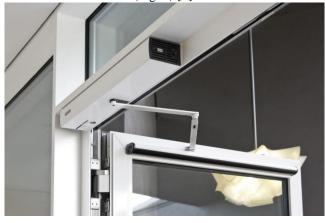
Fig. 2. Automatic drive for opening the access door.
