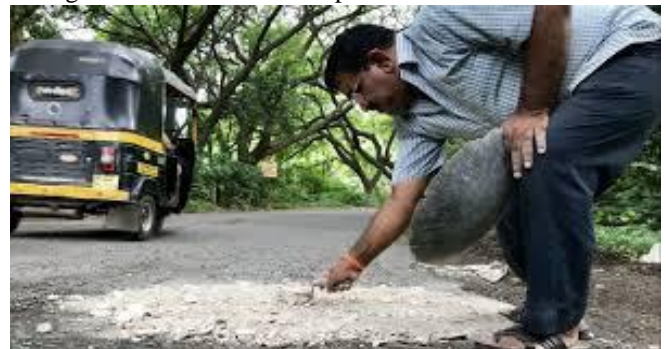
Fig 3 Improper roads leads to accidents
