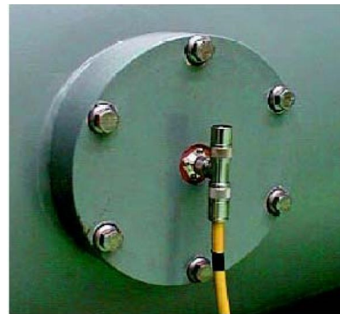
Fig 8. Sensor placed in dielectric window
