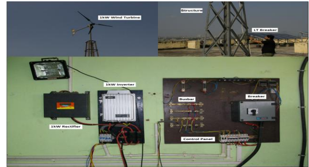
Figure.2.7. Installation of 1kW wind Turbine-Generator system at IEST roof top
