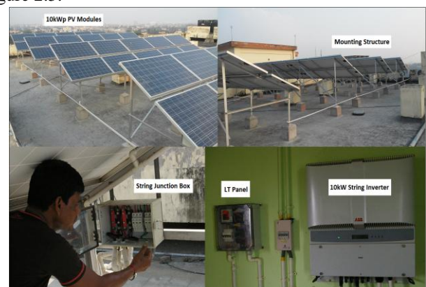
Figure.2.5. Installation of 10kWp solar PV power plant at IEST roof top
