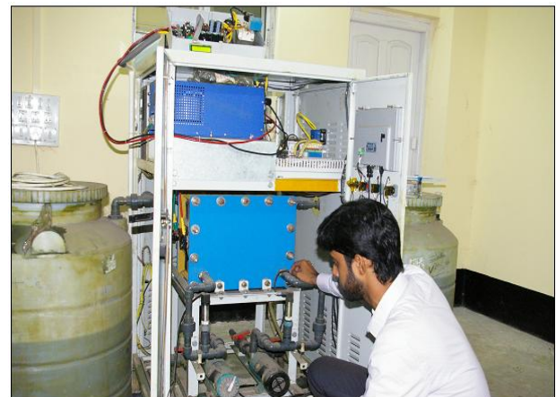
Figure.2.15. Installation of 1kW 6kWh VRFB storage at Microgrid Laboratory, IIST
