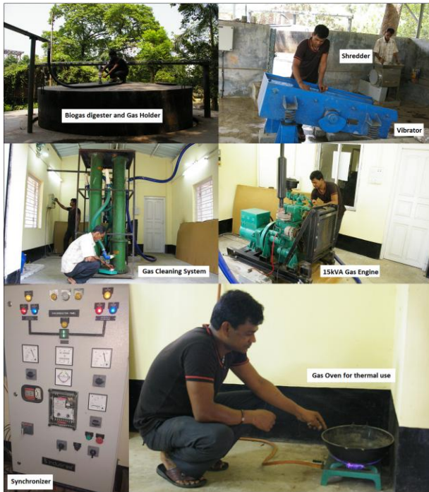
Figure.2.13. Installation of 15kVA biogas plant at IIST campus
