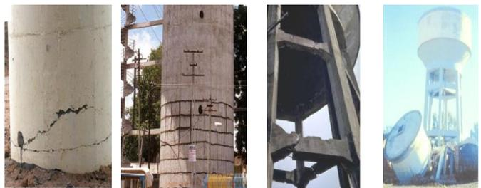
**Fig. 1.(a) Horizontal and diagonal circumferential cracks ,(b) vertical cracks ,(c) Flexural-shear failure is the repeated damage pattern of beams, (d) collapse elevated tank 1980 El- Asnam earthquake , Algérie**
