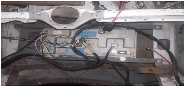
Figure.9. Final placement of motor controller
